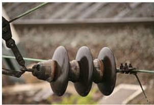
*"... The MTR Corporation has promised to replace a suspect batch of electrical insulators on the East Rail Line after a second fault in 10 days that caused delays for three hours during the evening rush... Services were hit from about 4pm after a faulty insulator in an overhead cable near Fanling station triggered a short circuit".* It took 10 days and 70 staff members to replace all the insulators from the installed batch at 65 critical locations.
