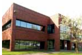
FLIR Systems, Portland
